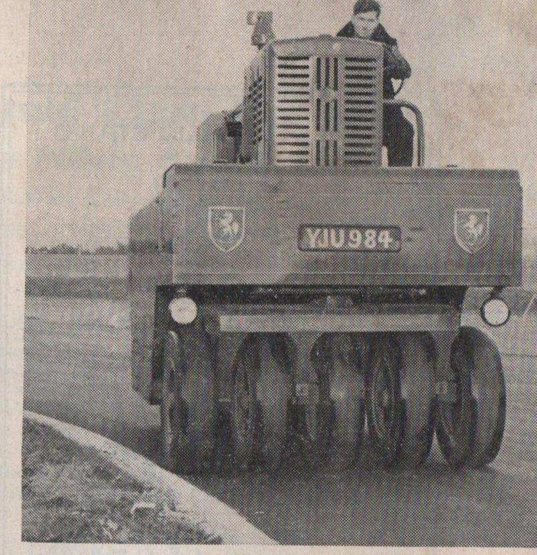
Slow drift round Madgwick. The 9-ton pneumatic-tyred roller working at a steady 3 m.p.h. and compacting the "carpet" on one of the fastest corners of the track.
